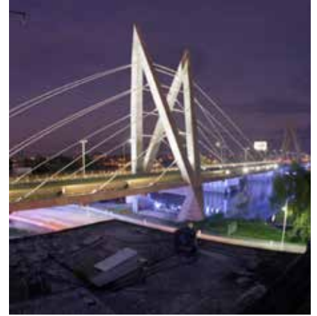
Grijalva Bridge Villahermosa, Tabasco
