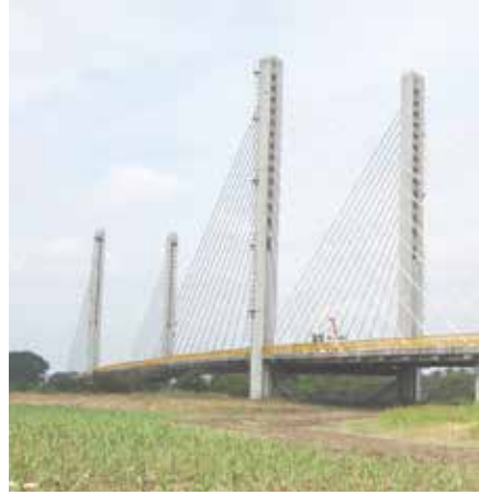
Papaloapan Bridge La Tinaja- Cosoleacaque Highway
