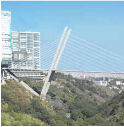
Vidalta Bridge Mexico City
