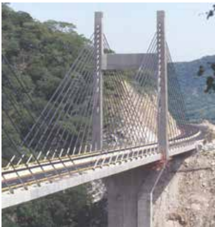
Quetzalapa Bridge México-Acapulco Highway
