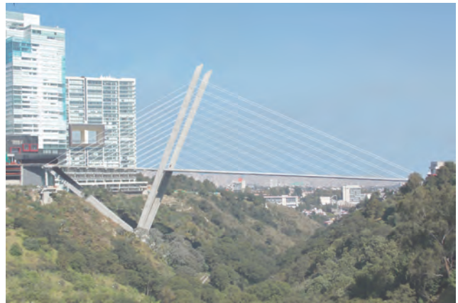
Vidalta Bridge , Mexico City
