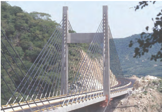
Quetzalapa Bridge, México-Acapulco Highway.
