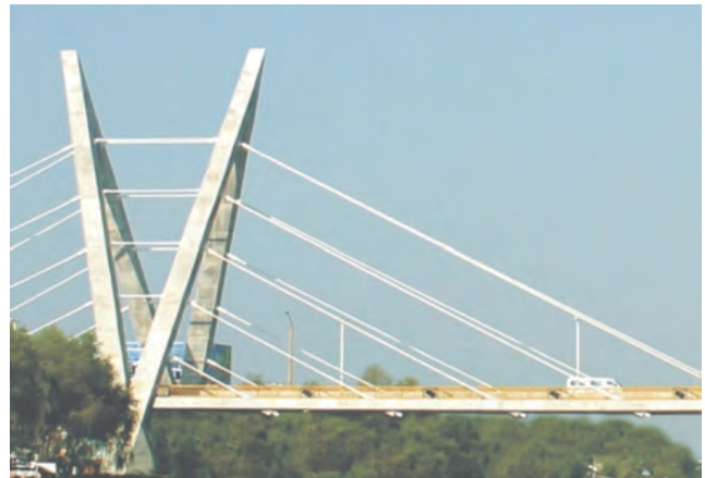
Grijalva I Bridge , Villahermosa, Tabasco
