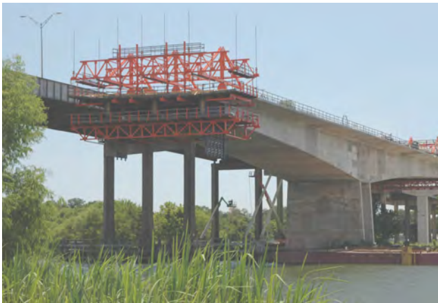
Puente "Trinity", Houston, Texas, USA
