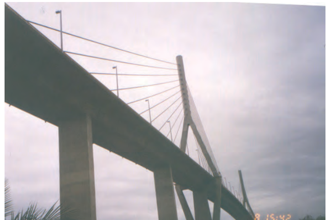
Tampico Bridge, Tampico, Tamaulipas
