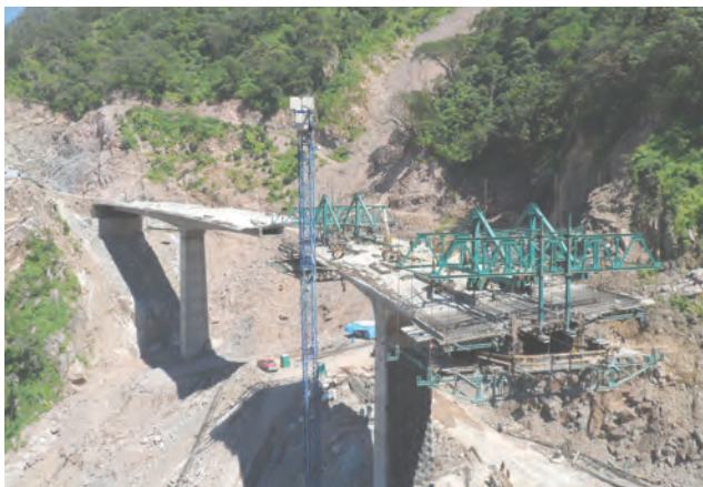
Platanito Bridge, Durango-Mazatlán Highway
