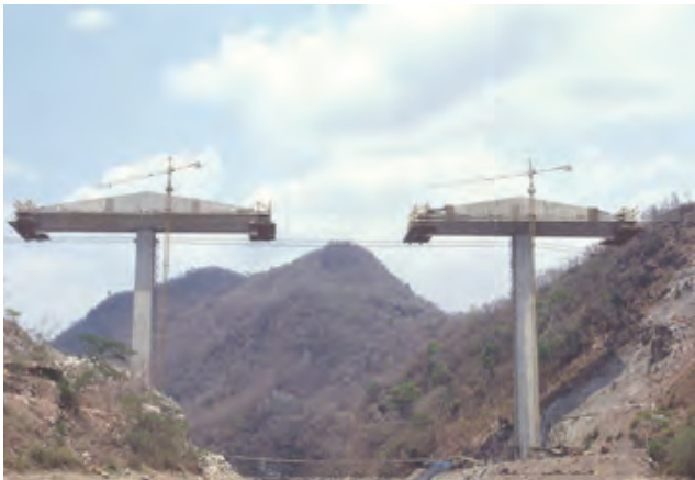
Papagayo Bridge, México - Acapulco Highway
