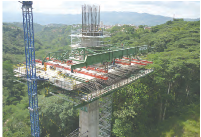
Carrera Novena Viaduct, Bucaramanga, Colombia
