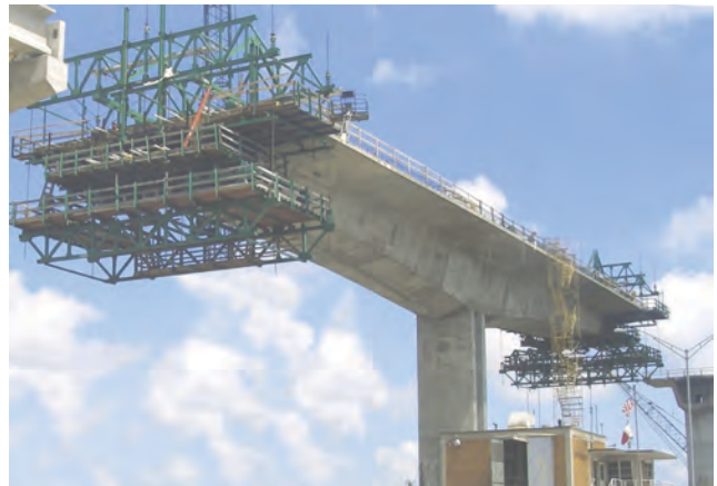
GIWW bridge, Texas, USA
