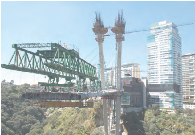
Vidalta Bridge, Mexico City
