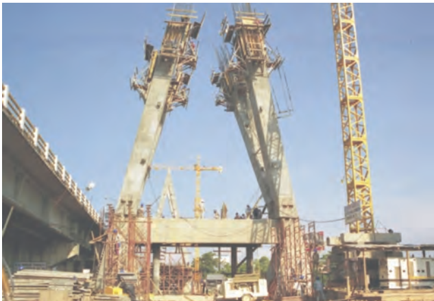
"Grijalva" Bridge, Villahermosa, Tabasco
