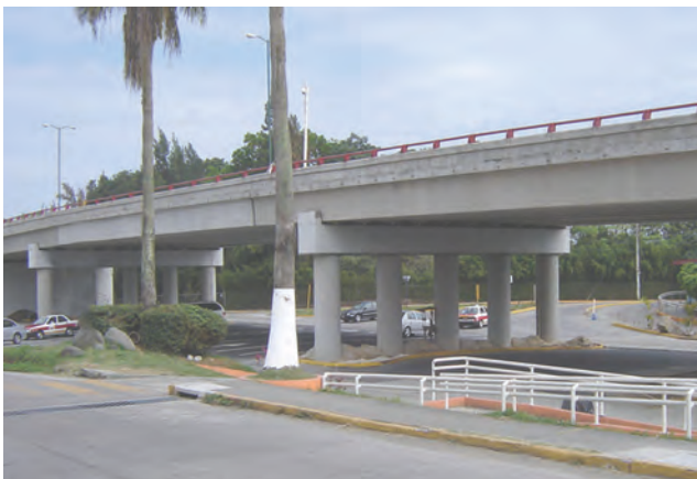
Chedraui Flyover, Córdoba, Ver
