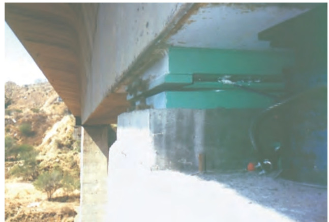
Atenquique II Bridge Guadalajara- Colima Highway
